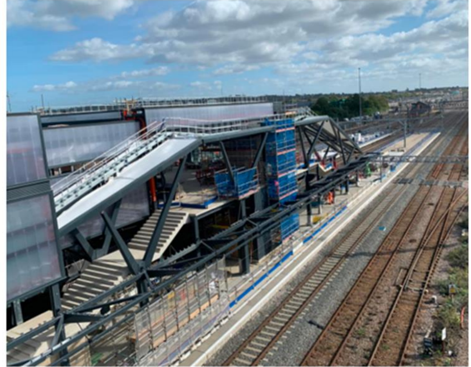
Stair and platform canopies
