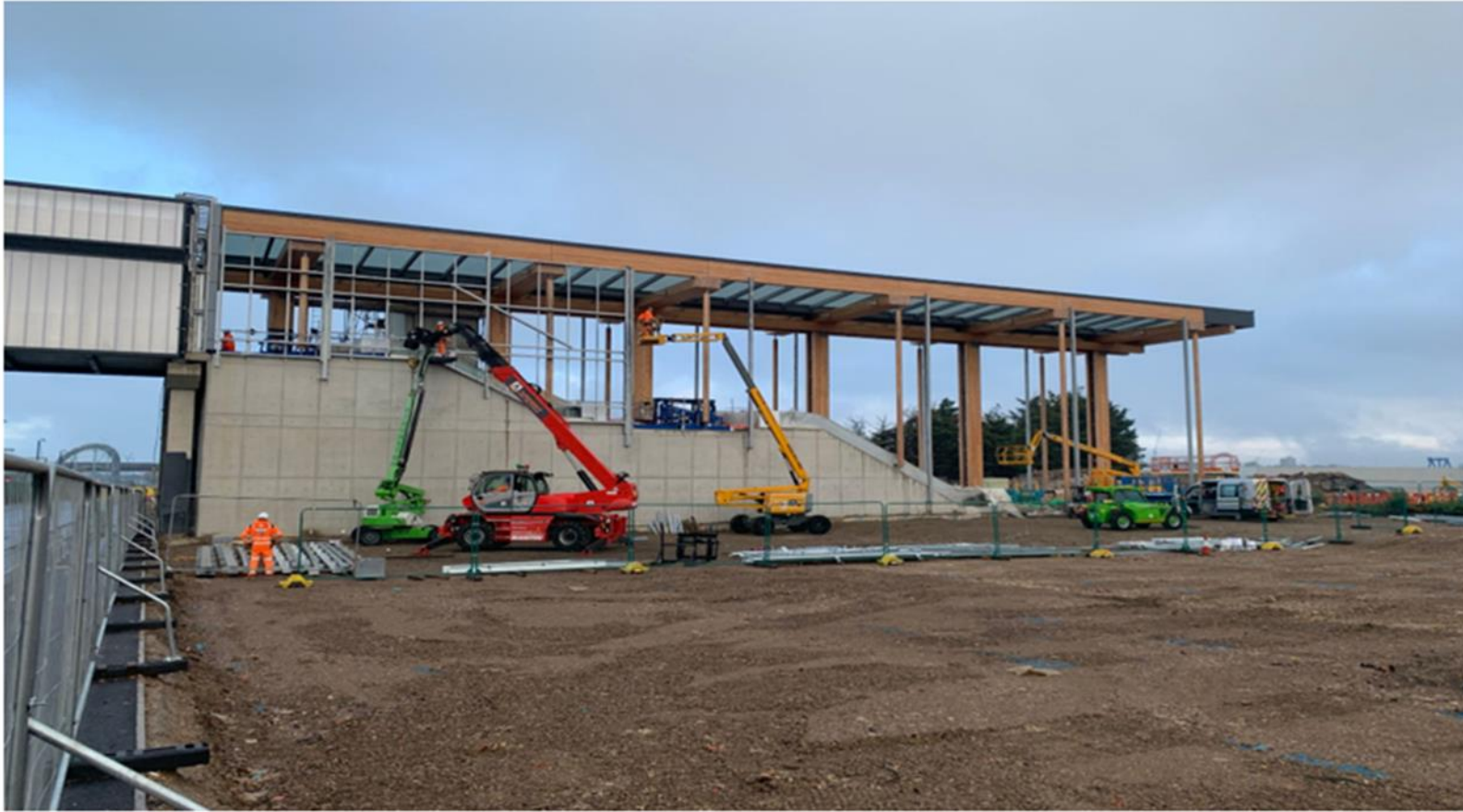
SEEB – South Elevation Hoarding
