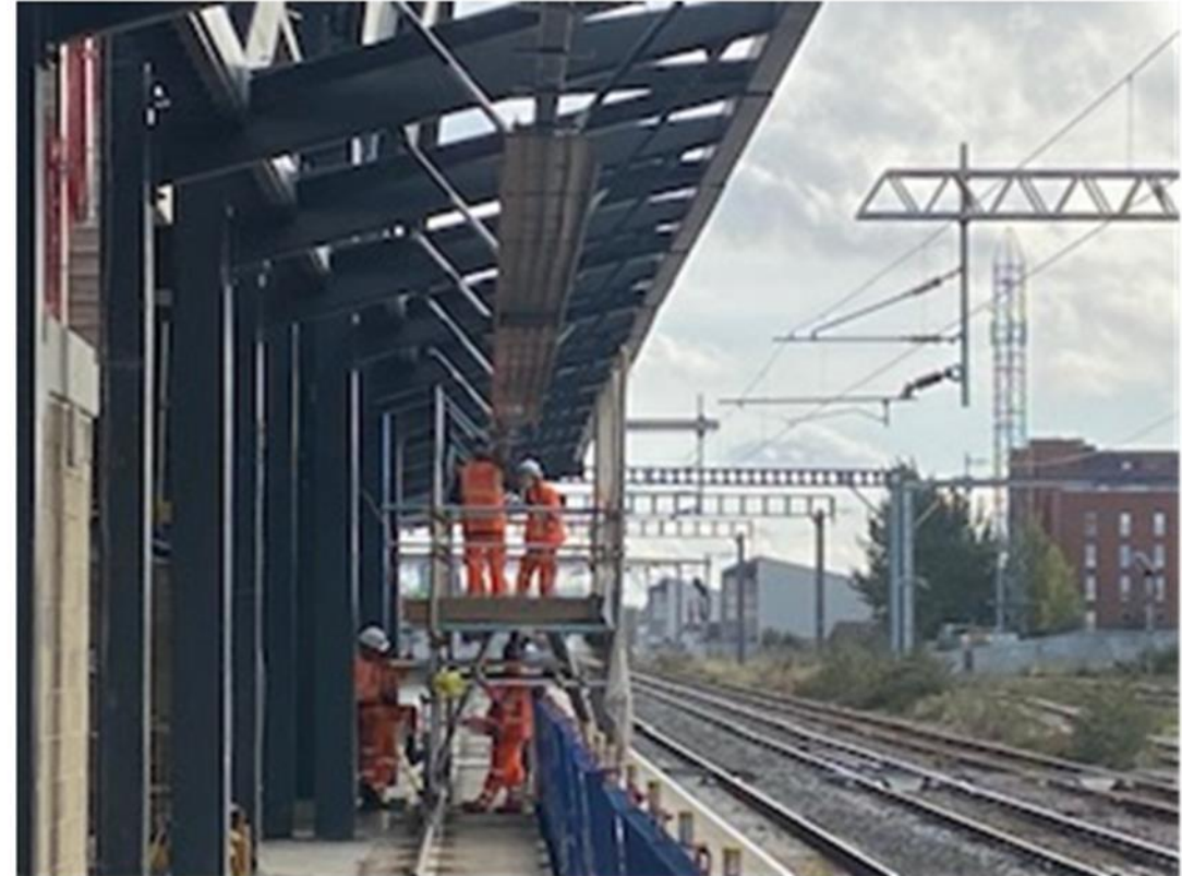
CMS installation to platform canopies
